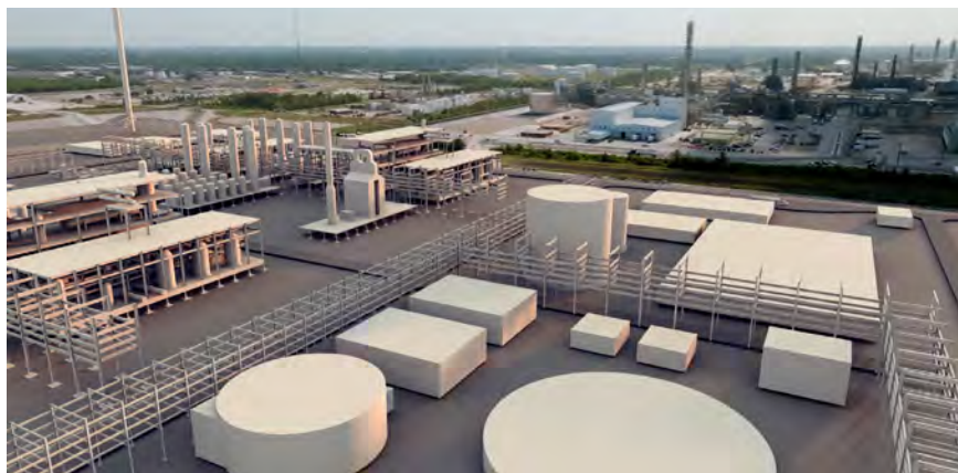
Baytown future hydrogen plant
